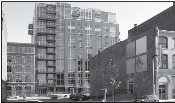
Channel Center, South Boston
